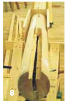
Figure 8—The excavation was prepared to receive a custom Sitka spruce Dutchman.
