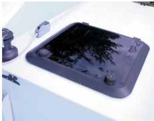
← Photo 7 —Clean off excess epoxy from the perimeter of the flange with the flat end of an 804 Reusable Mixing Stick. → Photo 8 —The finished hatch.
