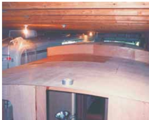
Left—The laminated cabin roof beams are in place.
