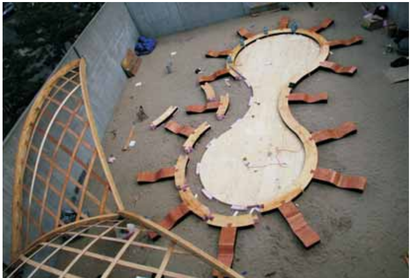
Figure 4—All sections were staged in place before they were bonded with epoxy thickened with a structural filler.
