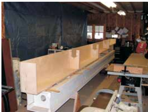
Dry fitting the tanks in the shop. The tanks are built of 1"-thick, 16-ply birch-faced plywood.
