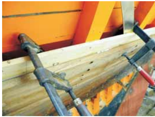
A "nibbed scarf" joint in the outer planking being glued together in place over the inner planking.
