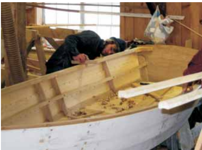
Traditional carvel or lapstrake are the construction methods used most often at The Apprenticeshop. Students here are working on a traditional lapstrake dory.
