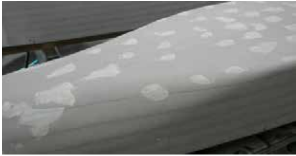
Figure 1.7 - Screw heads filled with drywall joint compound.
