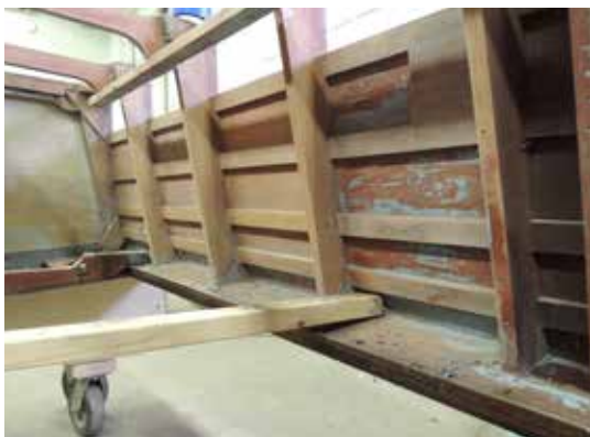
Rotted wood planks restored with new boards.
