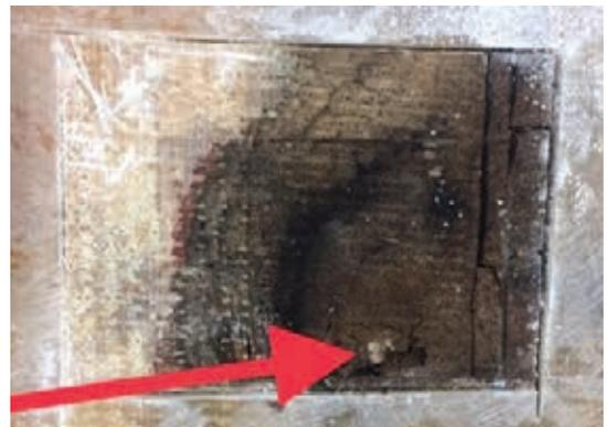
*You can see, with the skin removed on the underside of the hatch, the darker, more rotted wood around the column of epoxy putty.*
