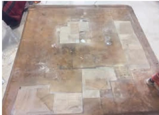
*Multiple areas had damaged core and needed replacement.*
