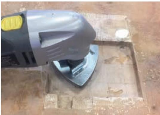
*Rotten and saturated core was cut away so replacement core could be installed. The area was then sanded with an oscillating saw.*
