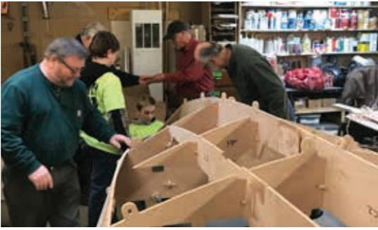
*Epoxy wetted T-pegs were driven into slots through the butt straps and into the parts being joined, ensuring vertical alignment as well as strength.*
