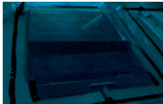
was placed on vacuum-tight sealing and infusion manifold positioning. Because of its higher viscosity, we weren't able to use the 105 System for the infused repair. We used our PRO-SET® INF 114/INF 226 Infusion Epoxy instead. Both methods successfully created similar cored laminates.
