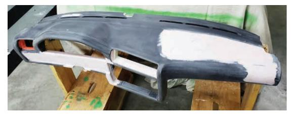
The insulation was faired in with 105/207 thickened with 410 Microlight Filler.
