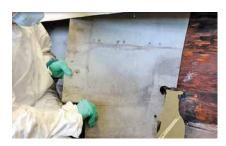
Removing the inner skin from the rotten plywood.
