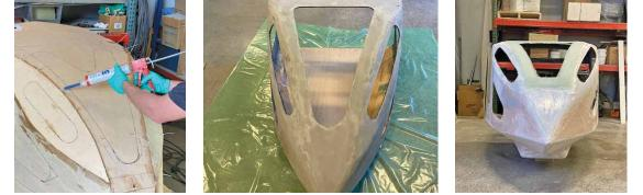
The outside of the shell was prepared with a grinder and orbital sander to smooth the corners, creating a radius edge for the fiberglass cloth. I applied one layer of 10 oz. fiberglass fabric over all of the plywood using WEST SYSTEM 105 Resin<sup>®</sup> and 206 Slow Hardener<sup>®</sup>. On the corners, I added a layer of 17 oz., 727 biaxial fiberglass tape.
