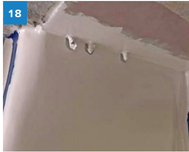
The surface was painted with flat white paint to finish the repair.
