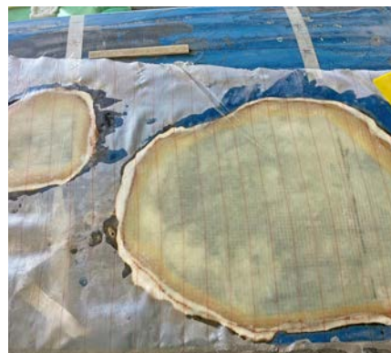
Fiberglass in place with release fabric.
